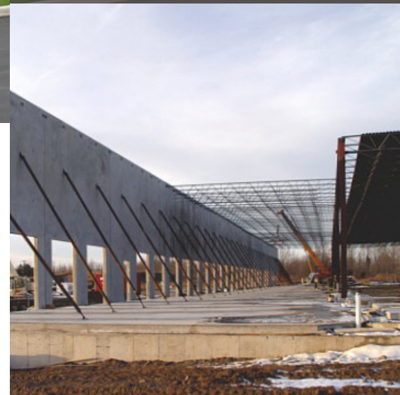
Concrete panels were site-cast, gently tilted up, and set in place to minimize construction time and maximize stability.
